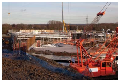
Construction of Olympic White Water facility, Broxbourne
